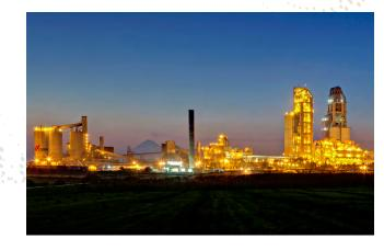
CEMEX cement plant in Prachovice (CZ) has a wide untapped waste heat potential amounting to ~16 MW. At the moment, it is not exploited in the facility, and it is rejected by means of water-cooling towers.
